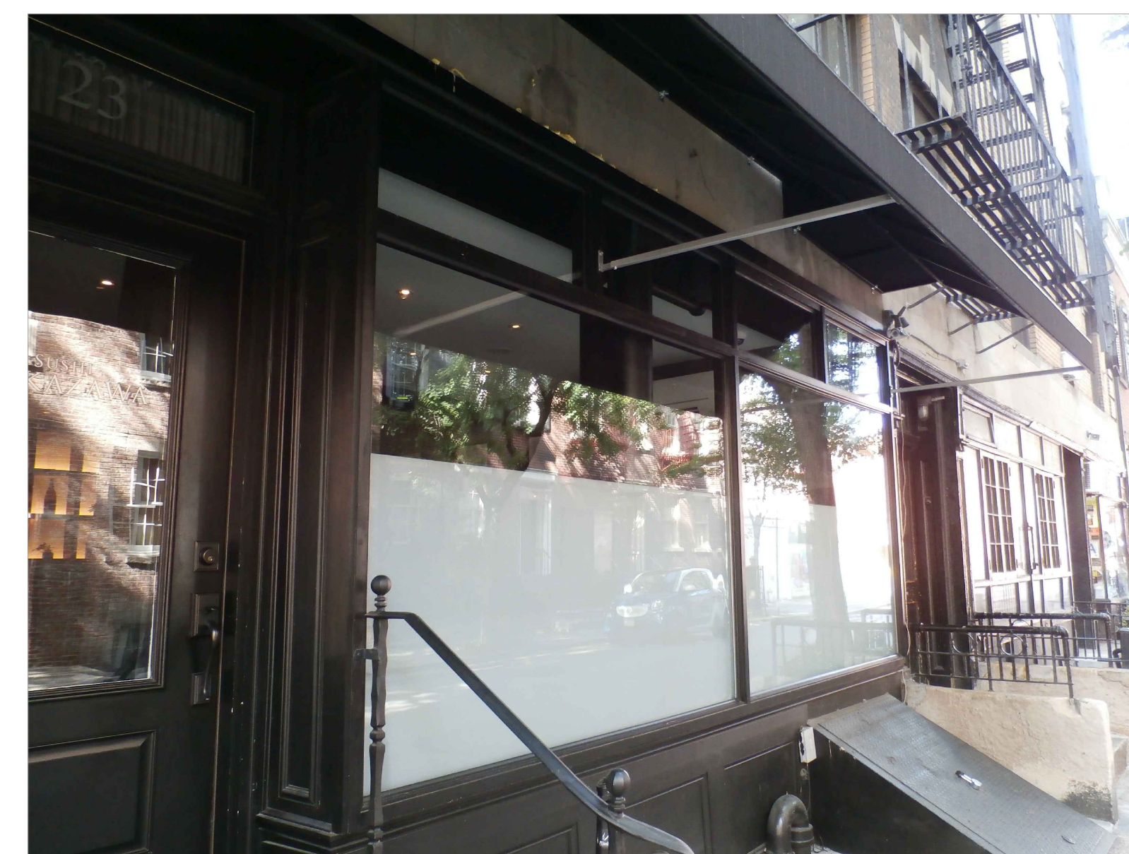
6 AS-BUILT: 2ND WESTERNMOST STOREFRONT
