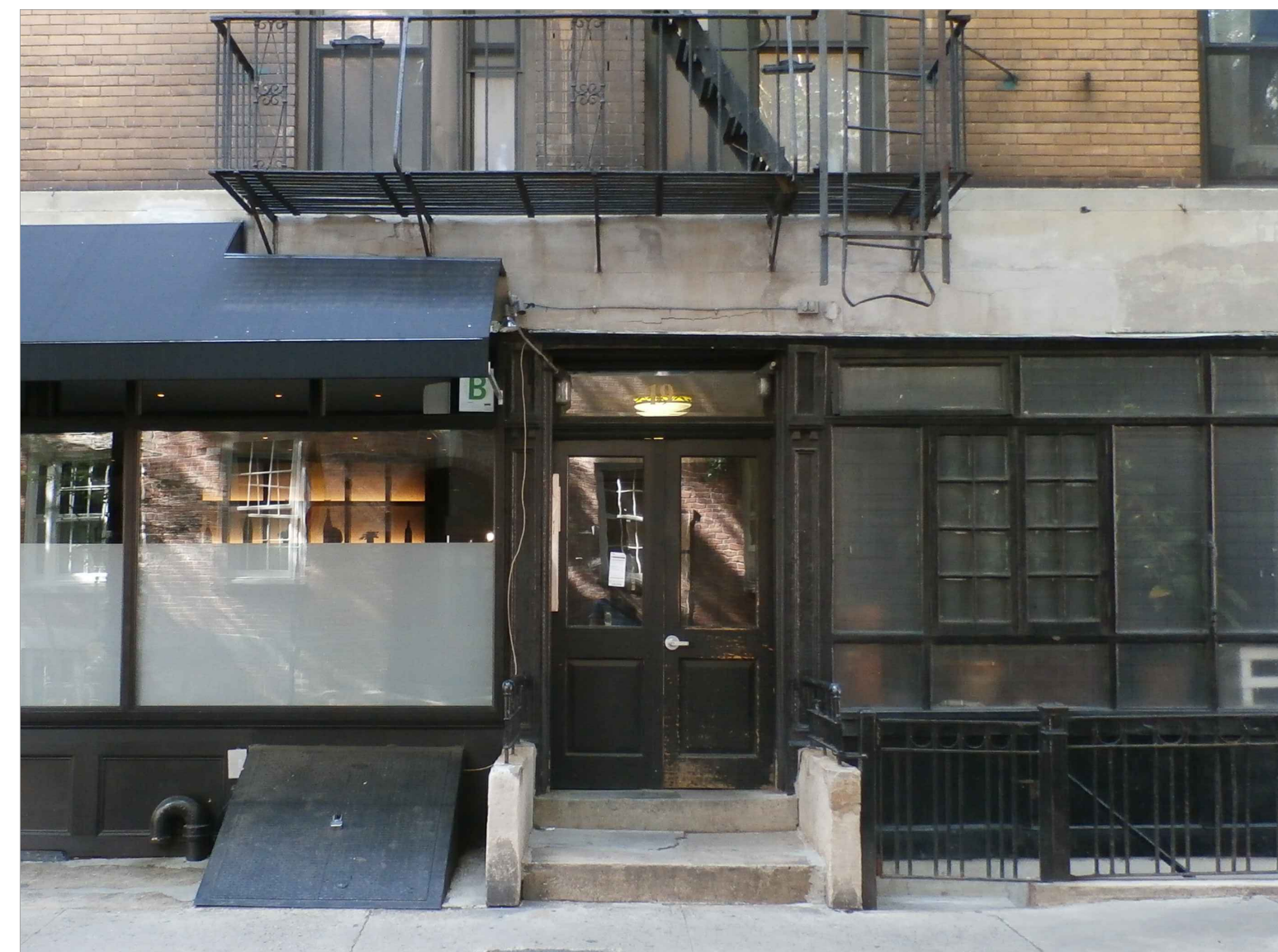
4 19-23 COMMERCE STREET CENTRAL ENTRANCE
