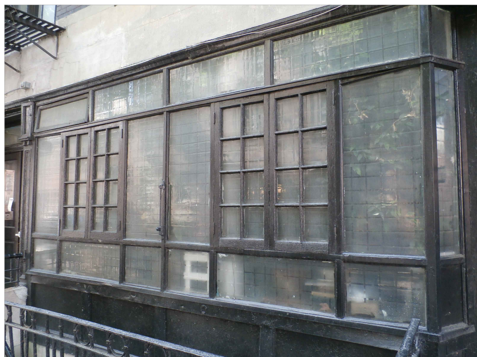
5 19 COMMERCE STREET HISTORIC WINDOWS
