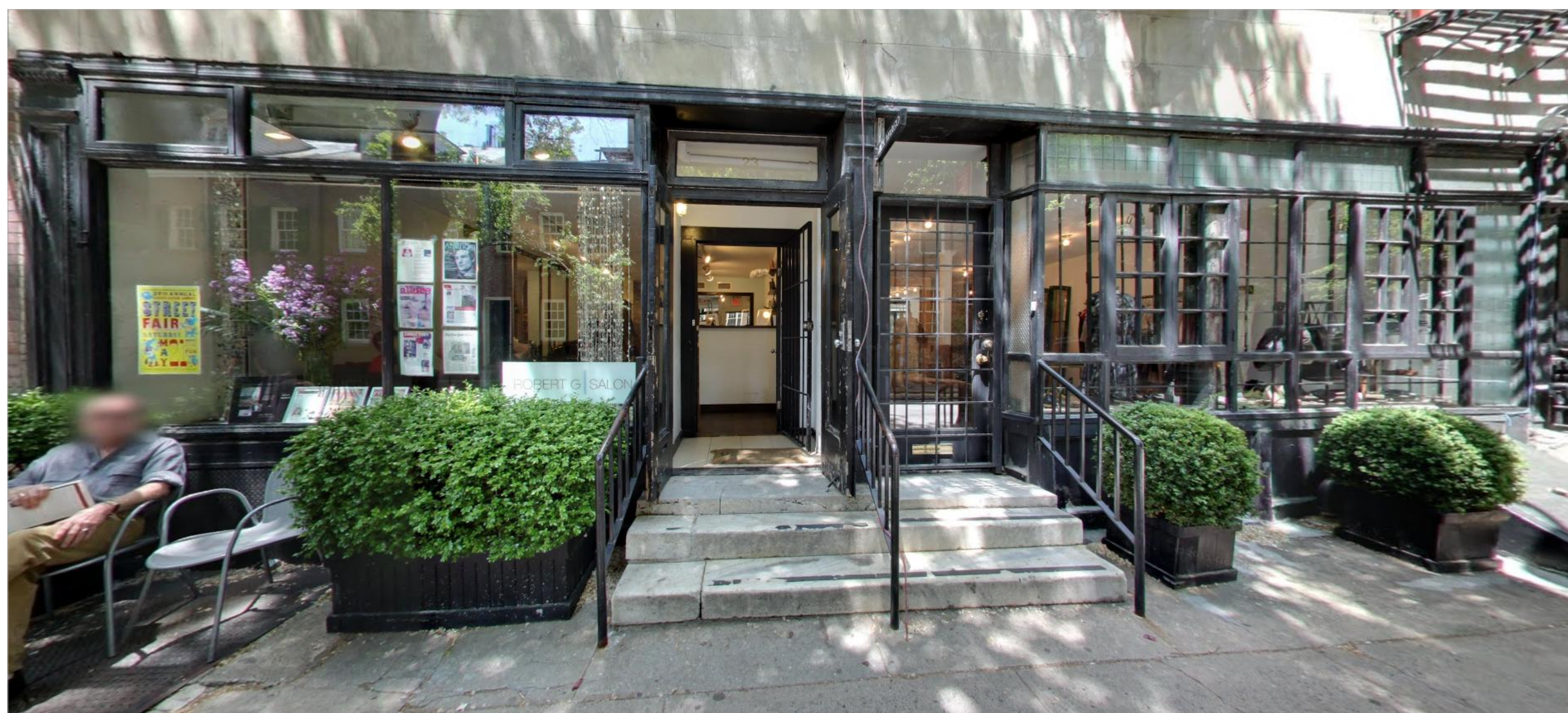
4 PRIOR-TO-CONSTRUCTION: 23 COMMERCE STREET STOREFRONTS (© 2011 GOOGLE STREET VIEW)
