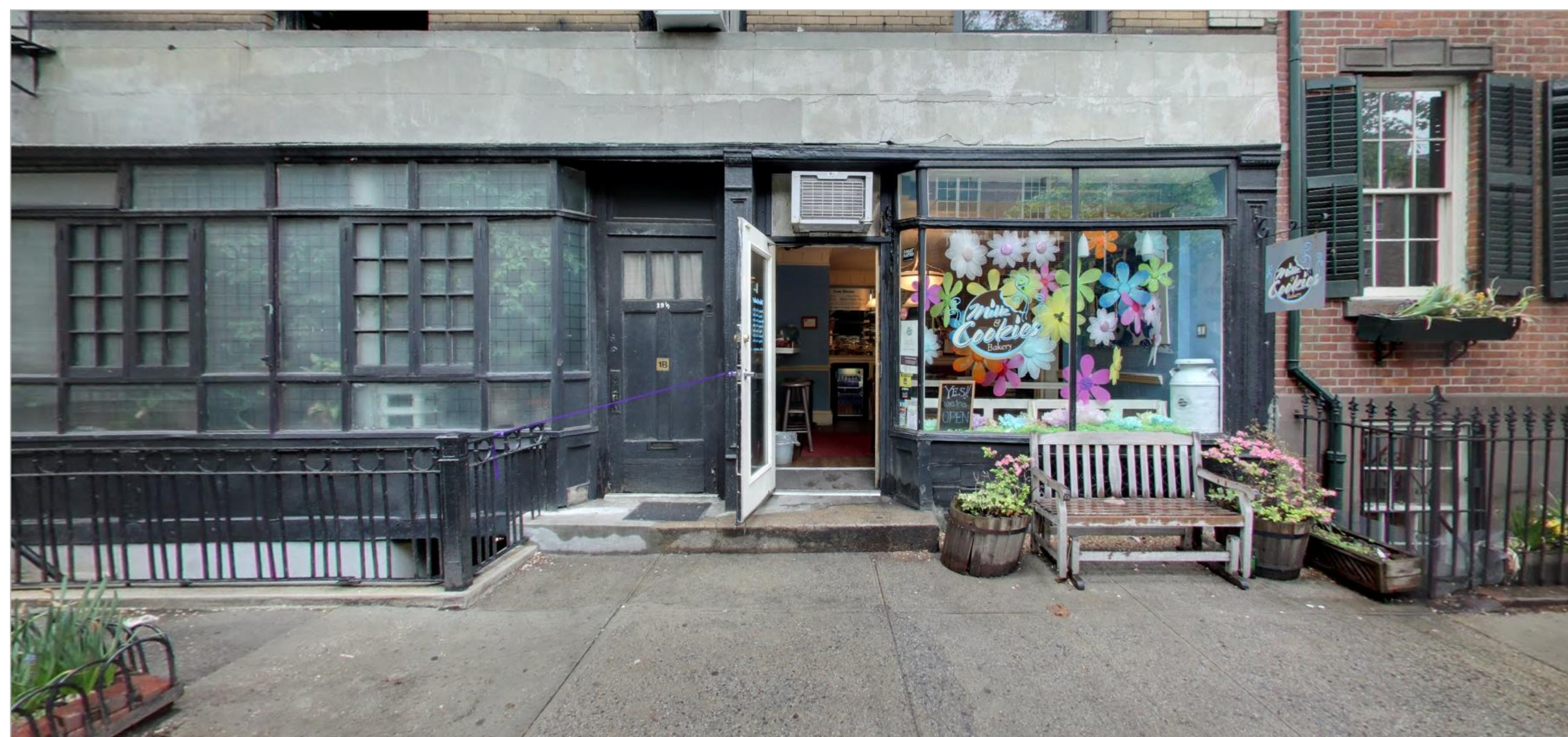
5 PRIOR-TO-CONSTRUCTION: 19 COMMERCE STREET STOREFRONTS (© 2010 GOOGLE STREET VIEW)
