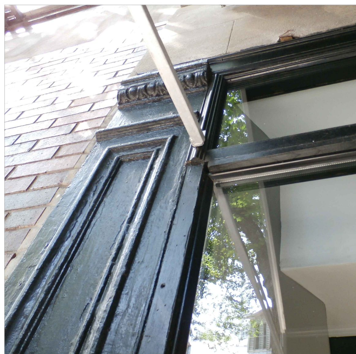
1 AS-BUILT: AWNING CONNECTION AT FRAMING
