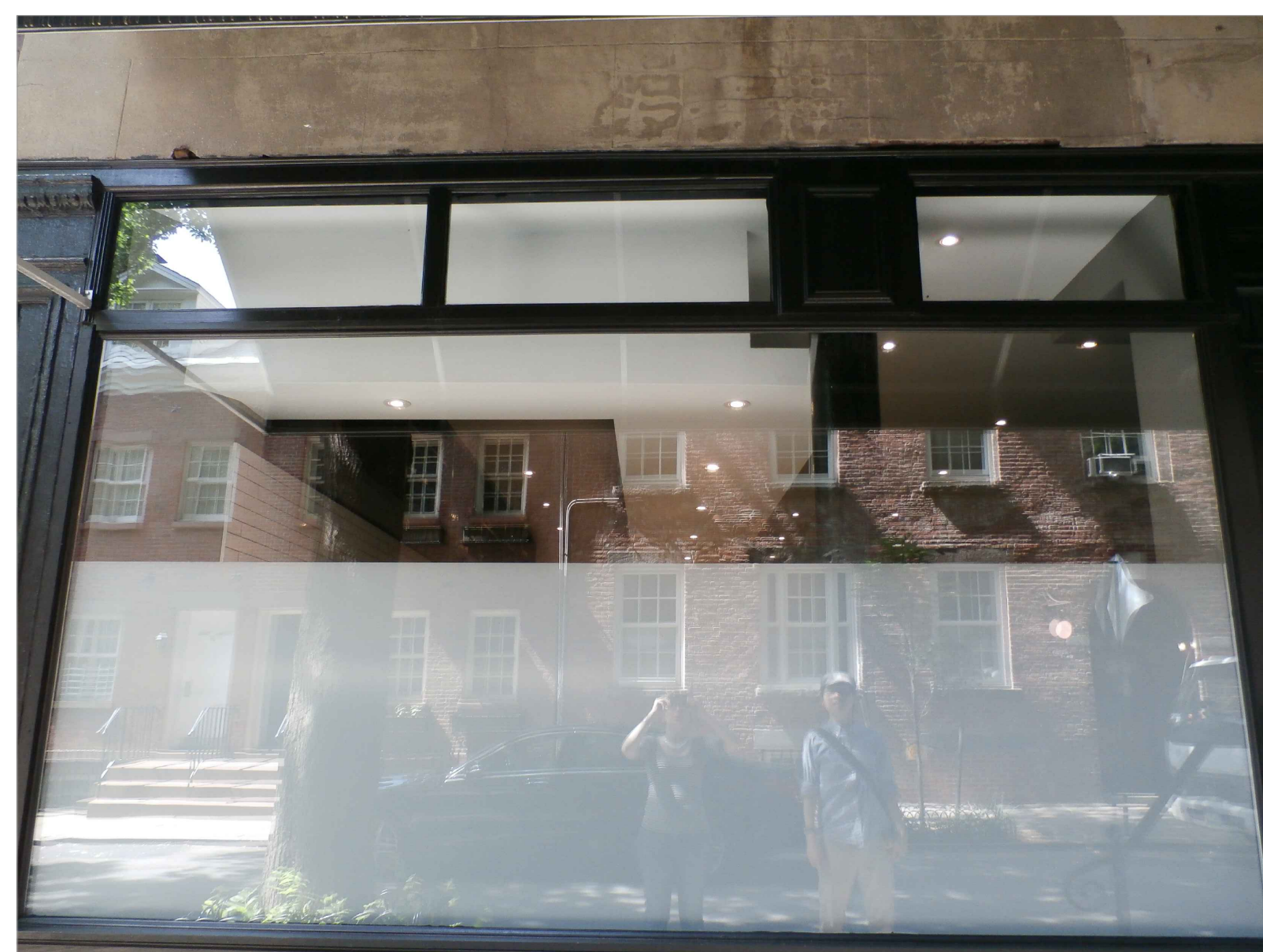
4 AS-BUILT: WESTERNMOST STOREFRONT
