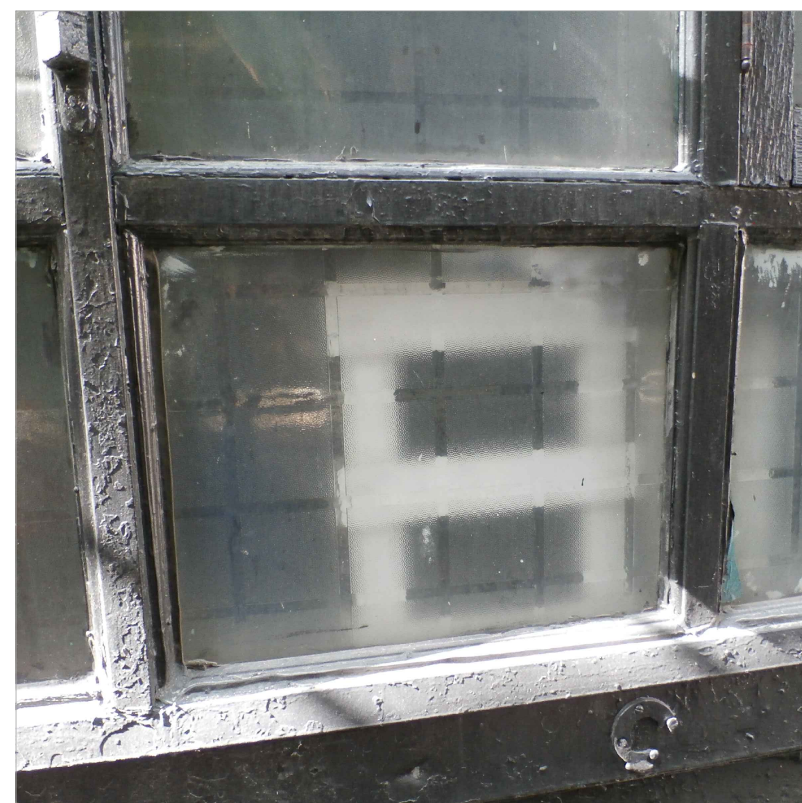
6 DETAIL: HISTORIC WINDOW PANE
