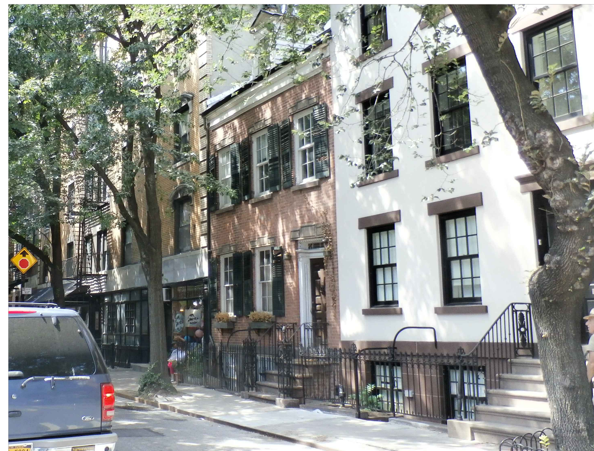
5 VIEW OF 19 COMMERCE STREET STOREFRONT: LOOKING WEST
